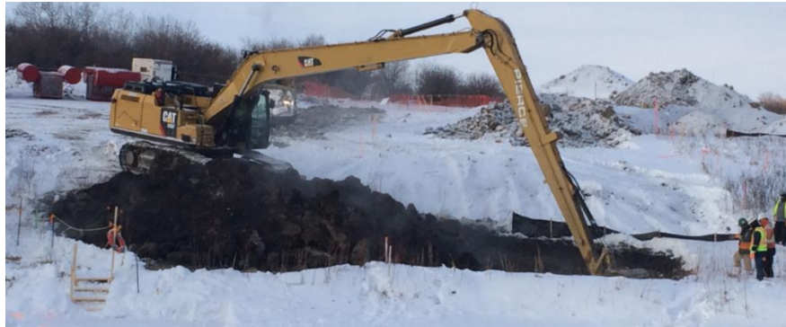
Pipe Stone Creek excavating west side
