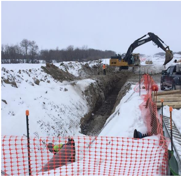
788 + 460 & 796 + 200 Excavating ditch for tie ins.
