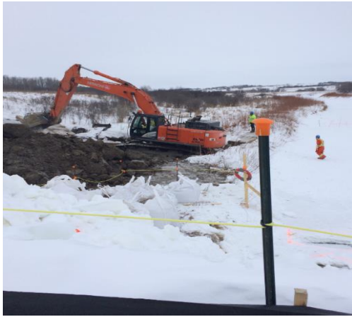
Excavating ditch line through the Pipestone Creek
