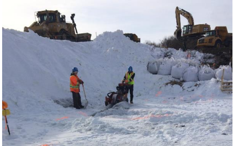
Pipestone Creek - Crew cutting line into the ice for the isolation
