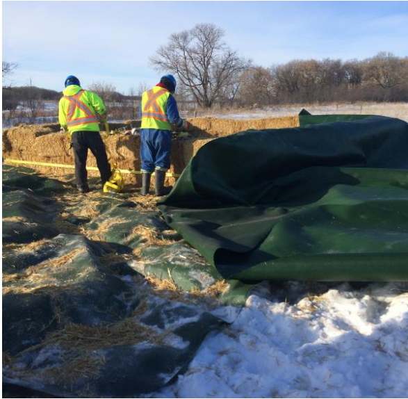
Crew setting up the straw bails and Geotextical membrane for the ditch water containment
