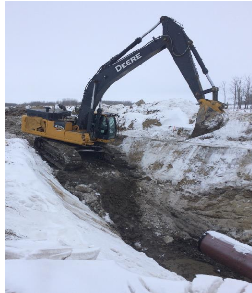
788 + 460 & 796 + 200 Excavating ditch for tie ins.
