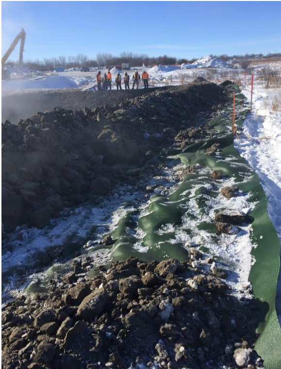
Pit constructed for Creek excavated material
