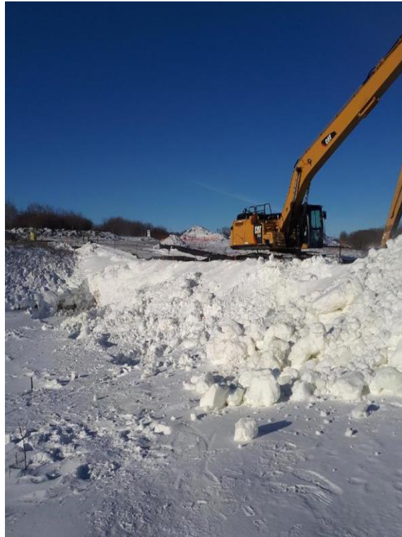
Cutting back the ice bridge to boundary on south side
