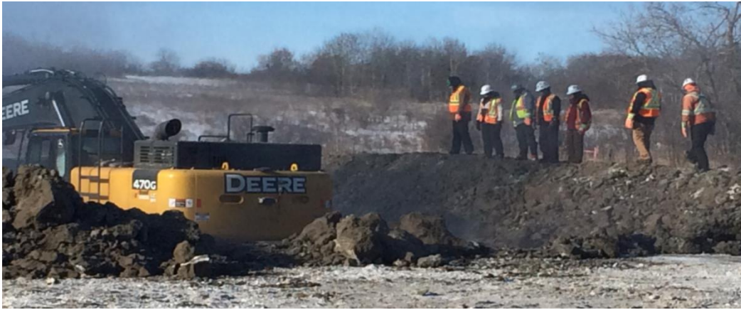
Excavating pit for Creek ditch material at the Pipestone Creek Archaeologist observing for items of interest in the soil
