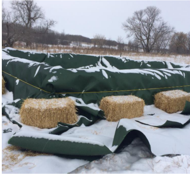
Crew setting up the straw bails and Geotextical membrane for the ditch water containment
