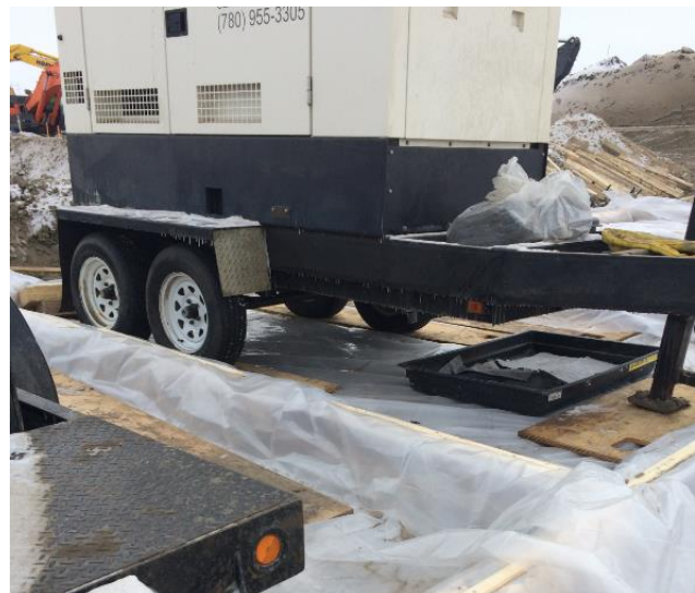
Hoses set across the Pipestone creek & Containment for the generators
