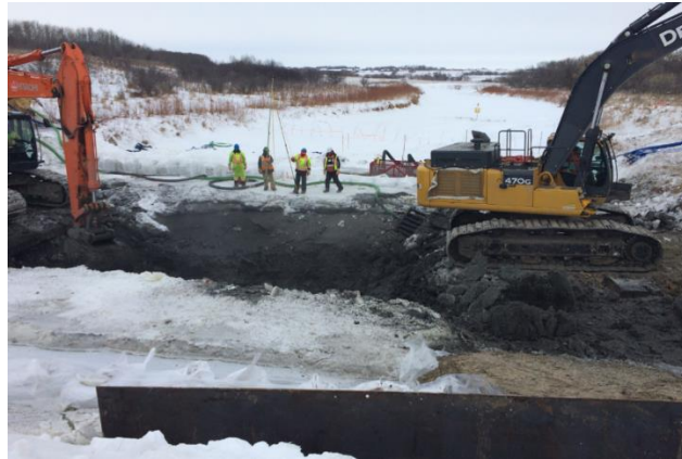
Excavating ditch line through the Pipestone Creek
