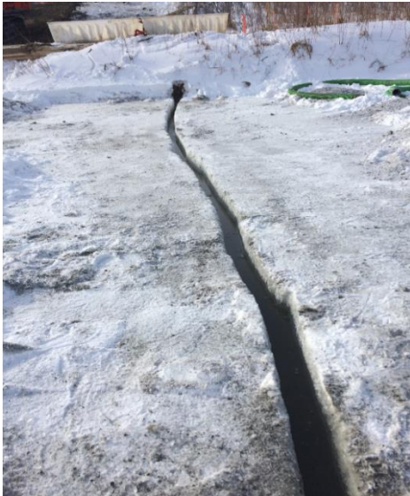
Pipestone Creek - Crew cutting line into the ice for the isolation
