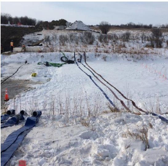
Hoses set across the Pipestone creek & Containment for the generators
